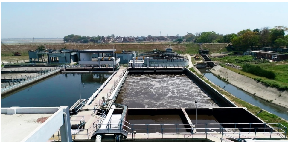
Sewage treatment using the SBR process
